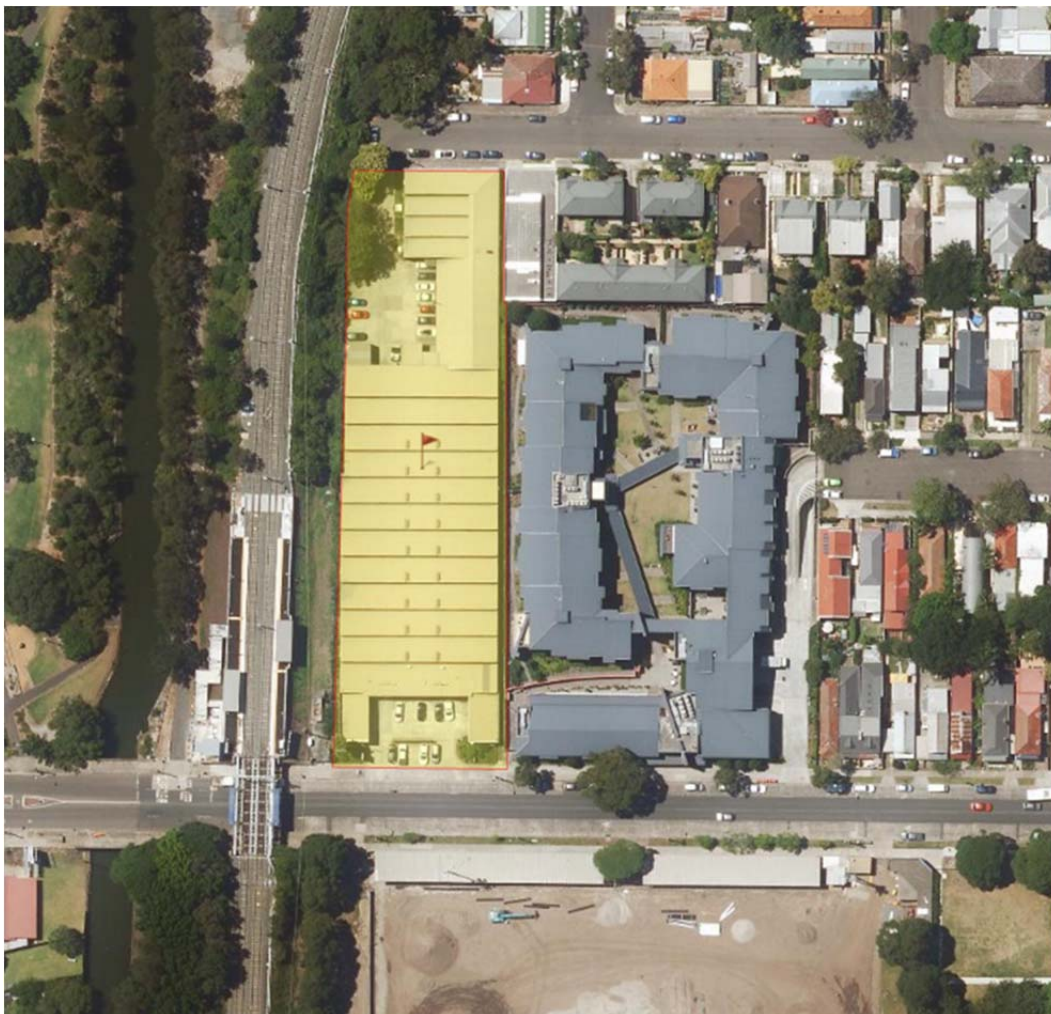
Figure 1: Aerial view of the subject site
